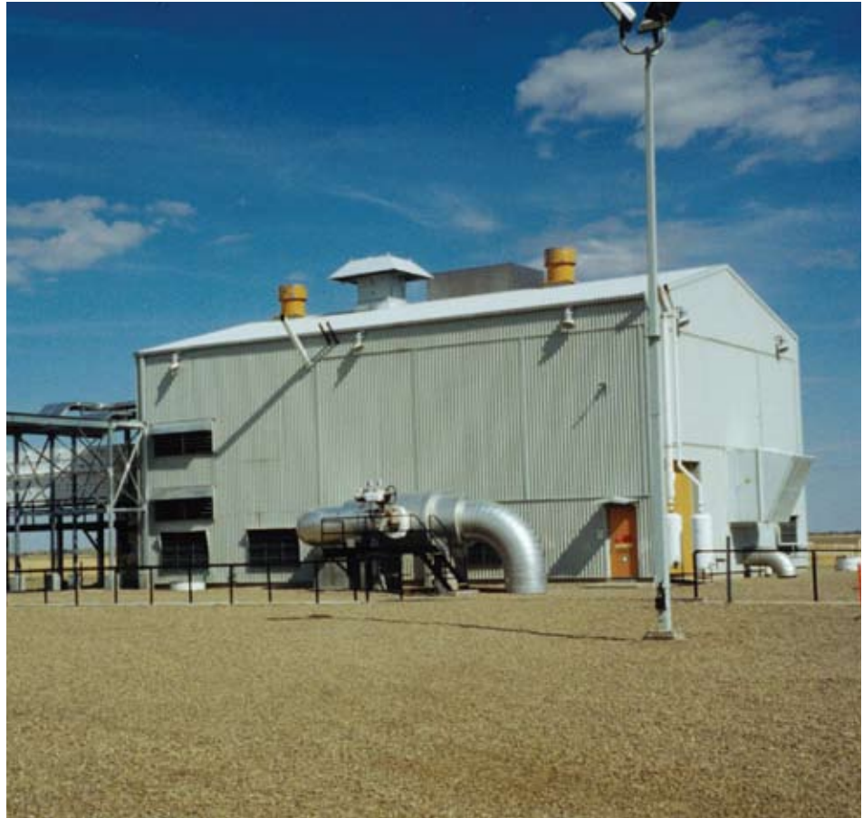
The MacKay River plant is key to Petro-Canada's bitumen extraction facilities.
