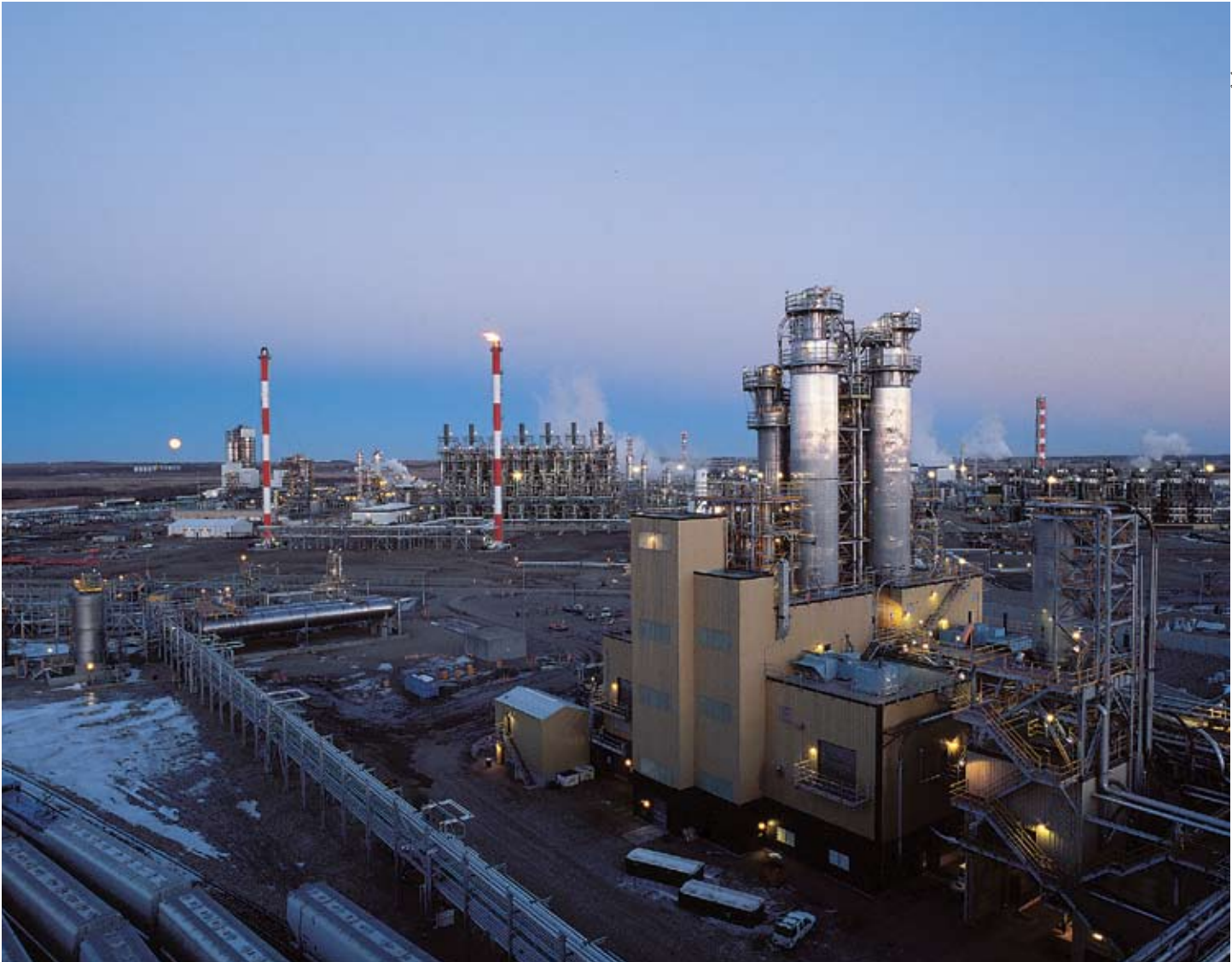
The NOVA Chemicals ethylene and polyethylene complex in Alberta is one of the largest in the world.
