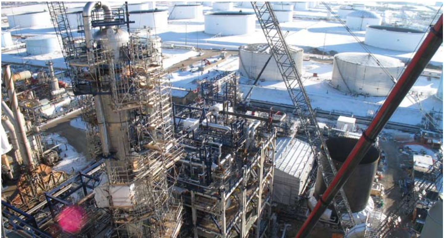
The Coker Fractionator Tower at the Petro-Canada Edmonton Refinery Conversion Project in 2007.
