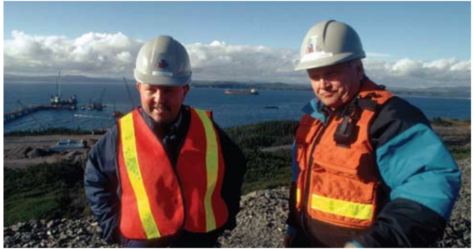
Paul Lovell, left, tours the Newfoundland Transshipment Terminal project site with Construction Manager Landis Krause in 1997.
